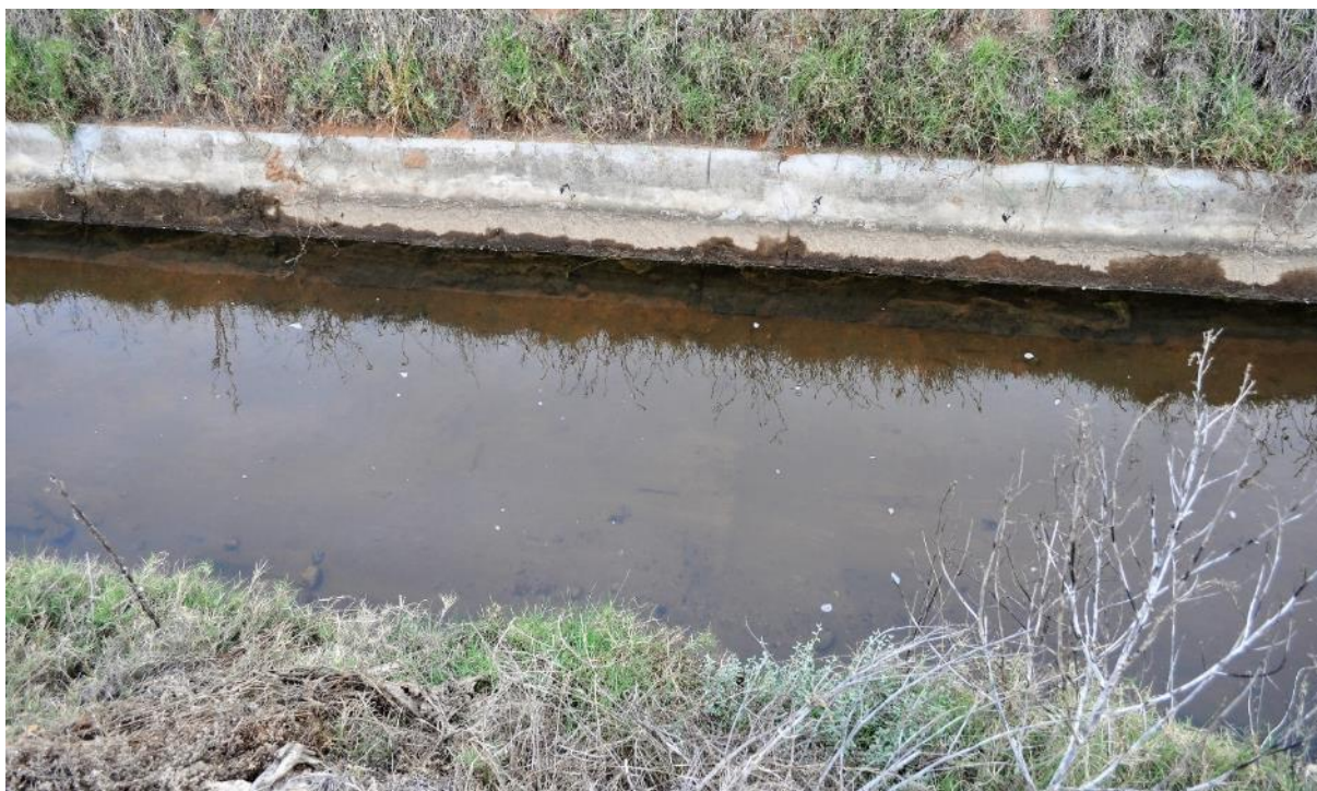
Figure 3.5 | Typical condition of concrete lining along the Clanwilliam Canal
