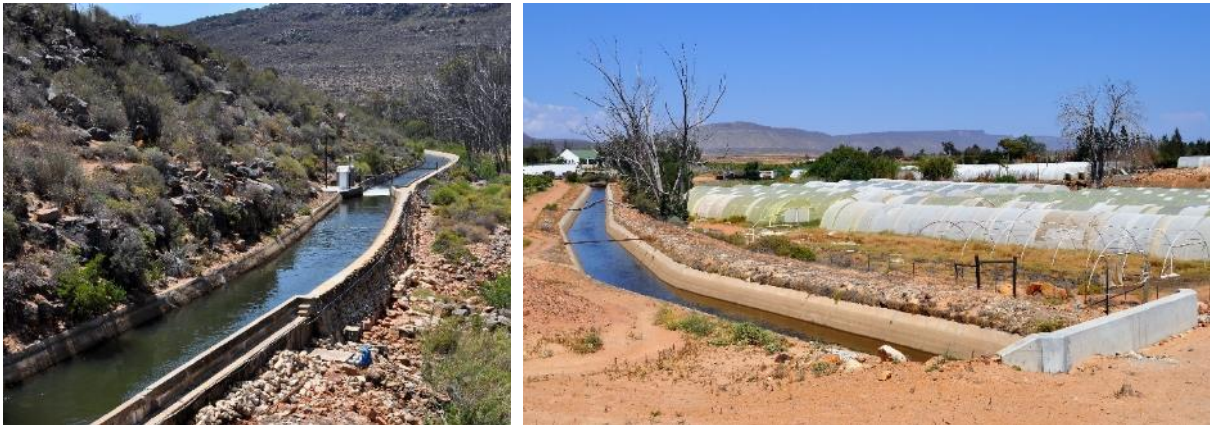
Figure 3.9 | The Lower Olifants Canal near Bulshoek Weir (left) and downstream
